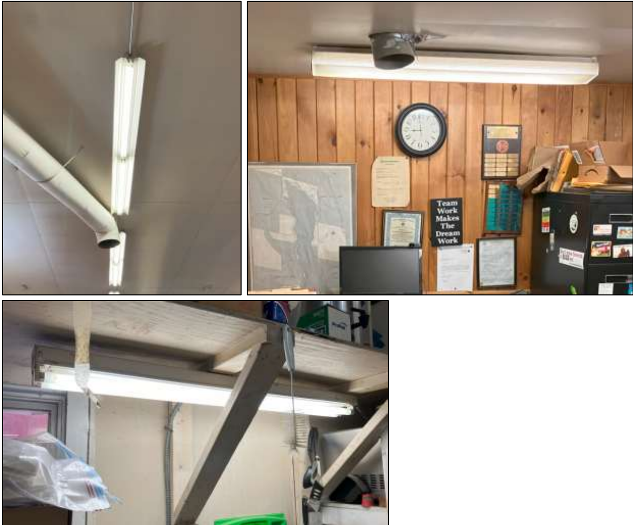
Clockwise from top left: Surface-mounted T8 fluorescent fixtures in apparatus bay, wraparound fluorescent fixture in office, strip fixture in kitchen
